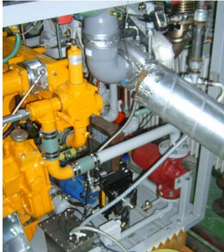
**Figure 5** Aactor !GT turbine acting only as a vacuum producer „Xhost Harvester ®“ on a very efficient natural gas CHP-plant of 90 kWe from Avesco. Together with the vacuum effect of “Xhost Harvester ®”, the CHP-plant reaches 40.1% (DIN) of electrical efficiency, which is very high for the engine size.
